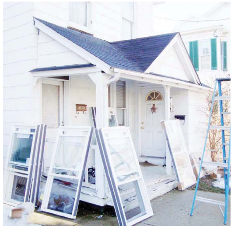
Workers prepare to install new windows at a neighborhood home.
